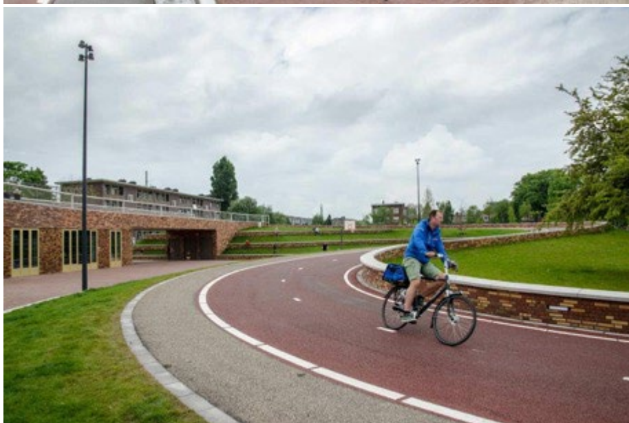
Slika 223 Dafne Schippersburg Bridge (Autor: NEXT architects, rudy uytenhaak + partners architecten, 2017.)
