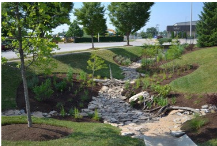
Slika 215 Kišni vrt uz prometnicu (Izvor: Unpacking Nature-based Solutions and Co-Benefits: A Primer )
